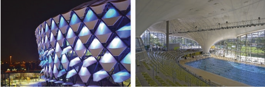
Fig. 2.2 Two examples of tensile structures in large-scale constructions. Left: Glass/PTFE membrane panels for external shading at Hazza Bin Zayed Stadium (© Christoph Paech/schlaich bergemann partner). Right: Membrane roof of Olympic Aquatic Centre, Munich (© Michael Zimmermann/schlaich bergemann partner)
