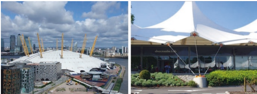
Fig. 2.5 Example of a boundary-tensioned structure: Millenium Dome (O2 Arena), London (left) [16]; McArthurGlen Designer Outlet Village; architecture: Richard Rogers; engineering and fabrication: Buro Happold, Tensys Ltd., Architen Landrell (right)
