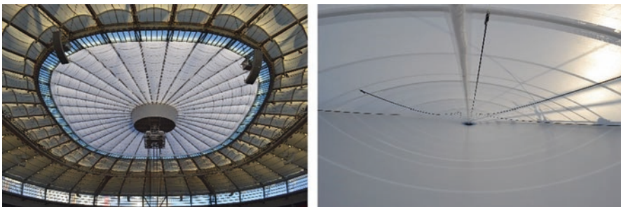
Fig. 2.7 Example of a pneumatic structure with cushion realized in PTFE-coated PTFE weave (left) and internal view of inflated cushion (right). BC Place Stadium, Vancouver, CA (© Christoph Paech/schlaich bergemann partner)
